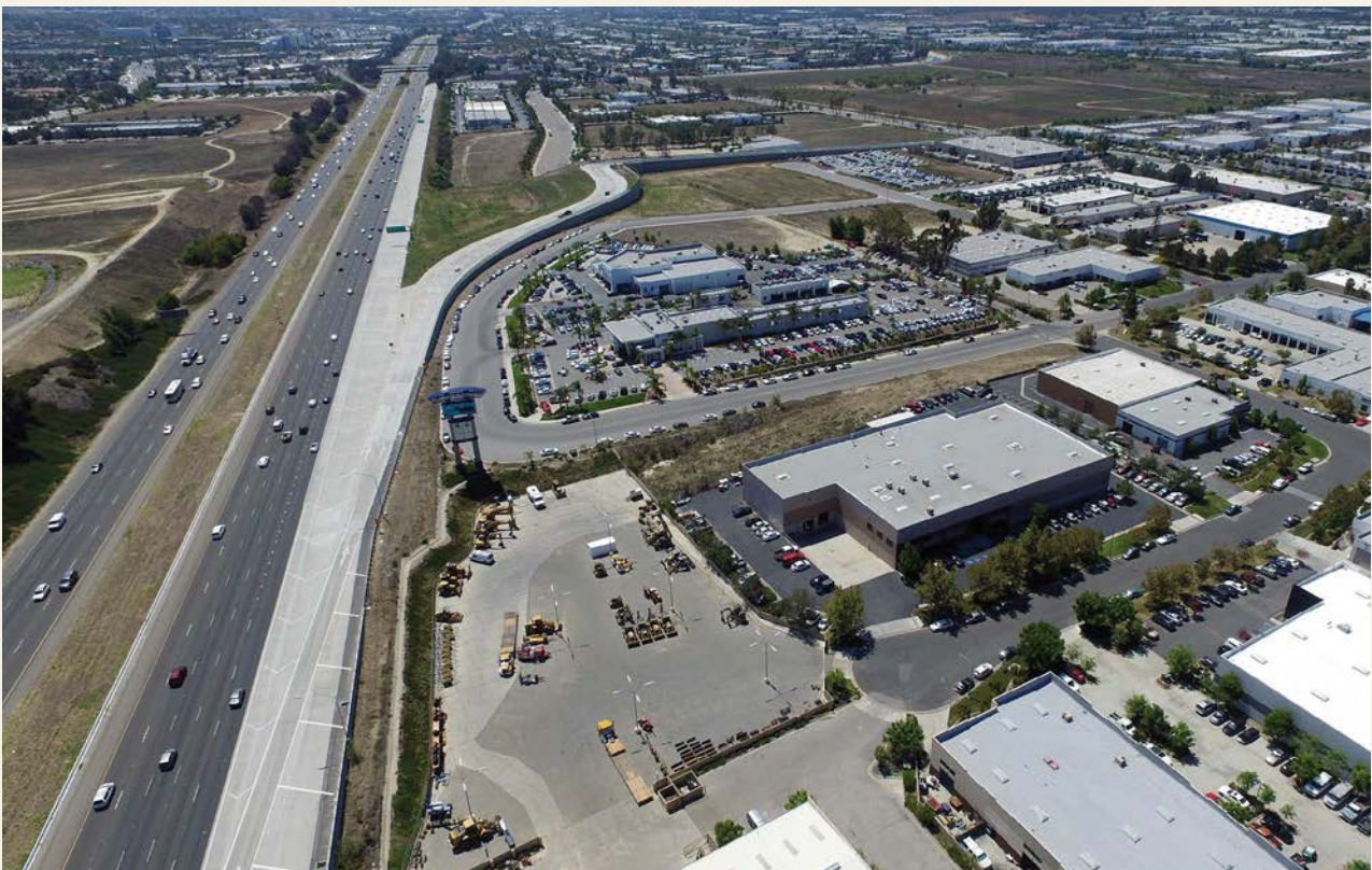
French Valley Parkway off-ramp project
